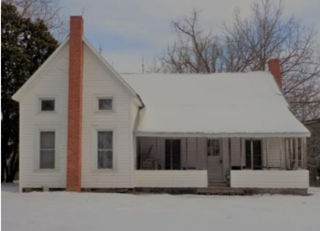
c.1890s house at Yost-Ketner Farm, (RW2172) façade and front yard, looking east
