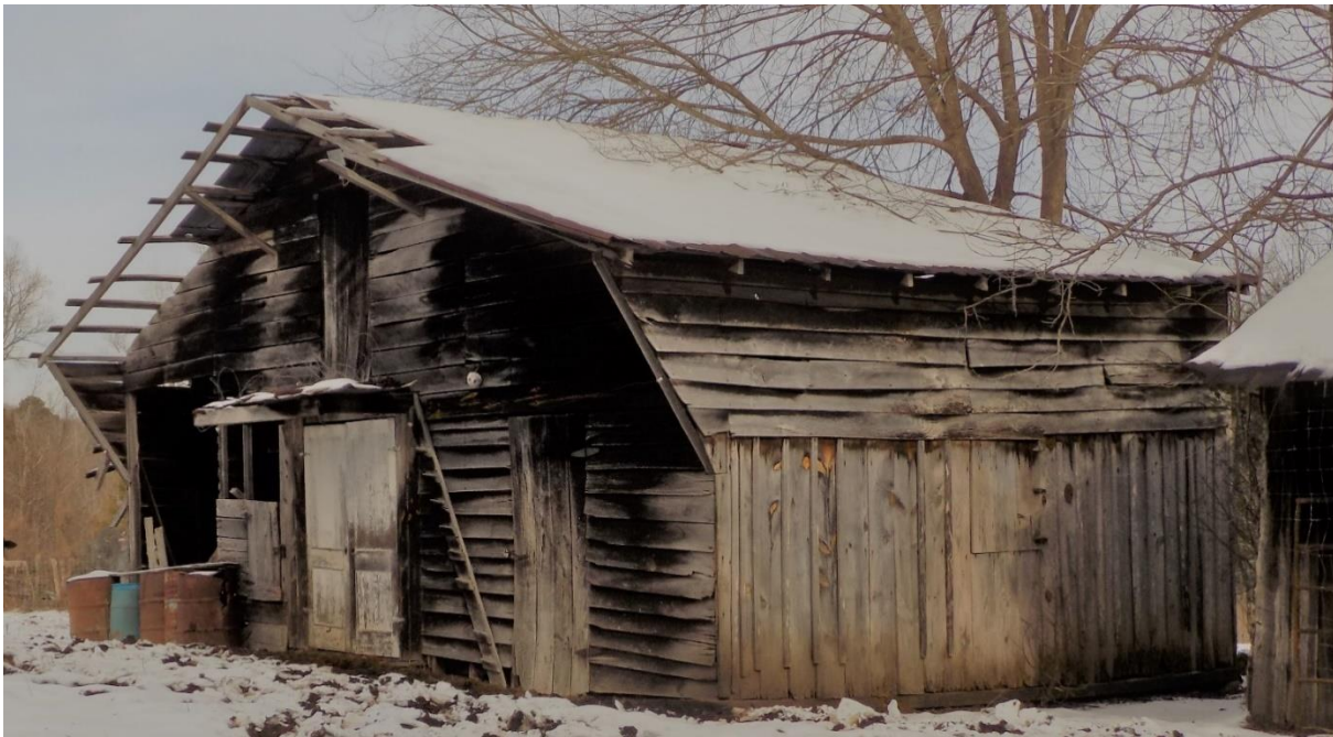
Granary located to the north of the car shed, looking north
