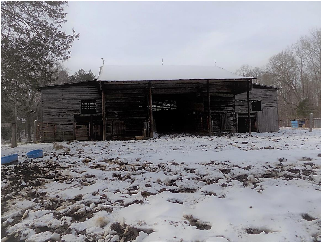
Front of the double-crib barn looking west
