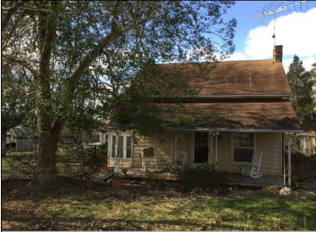
Sides-Carter House façade, looking west
