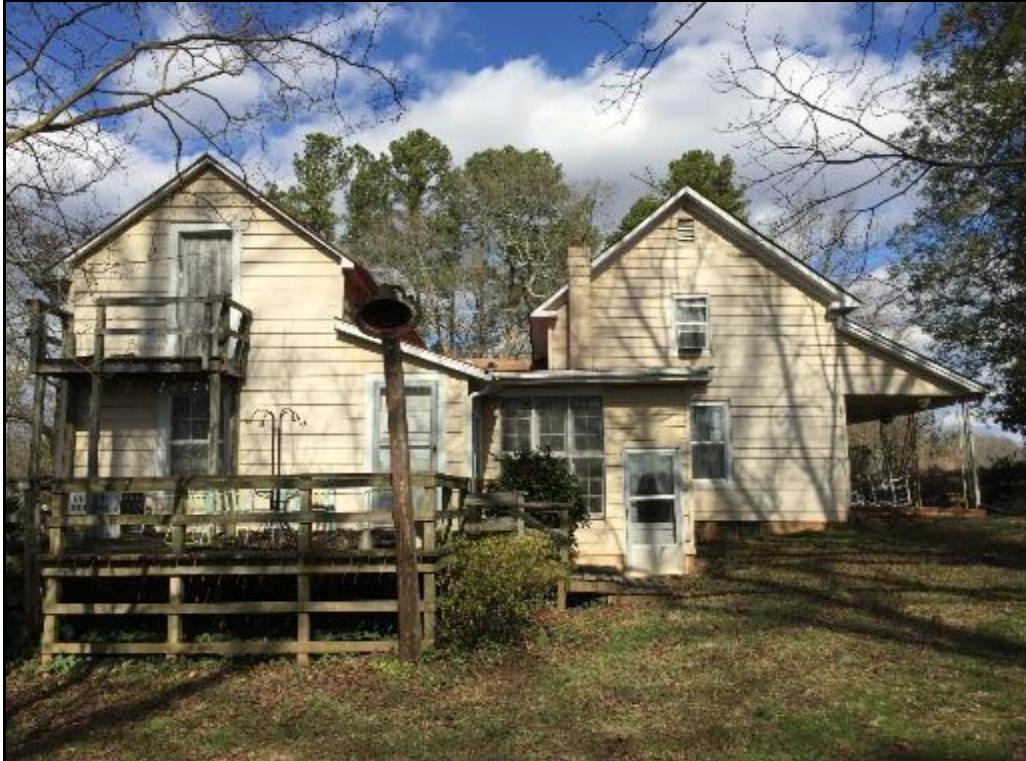
Rear additions to the Sides-Carter House, looking north
