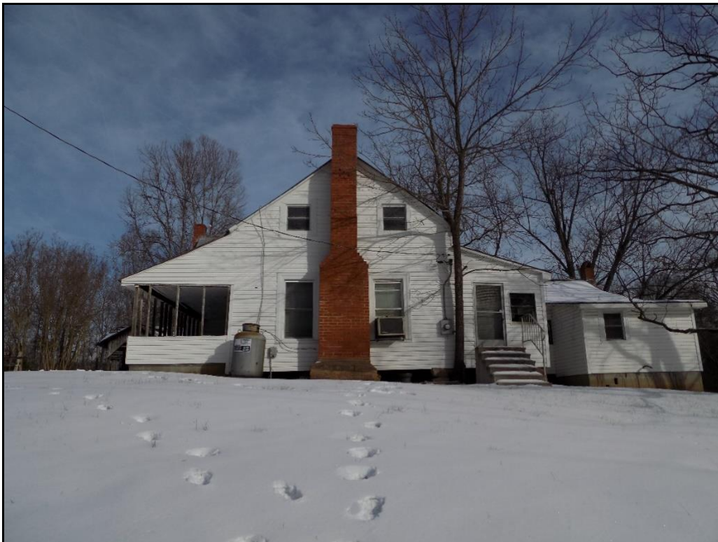
South elevation of main house
