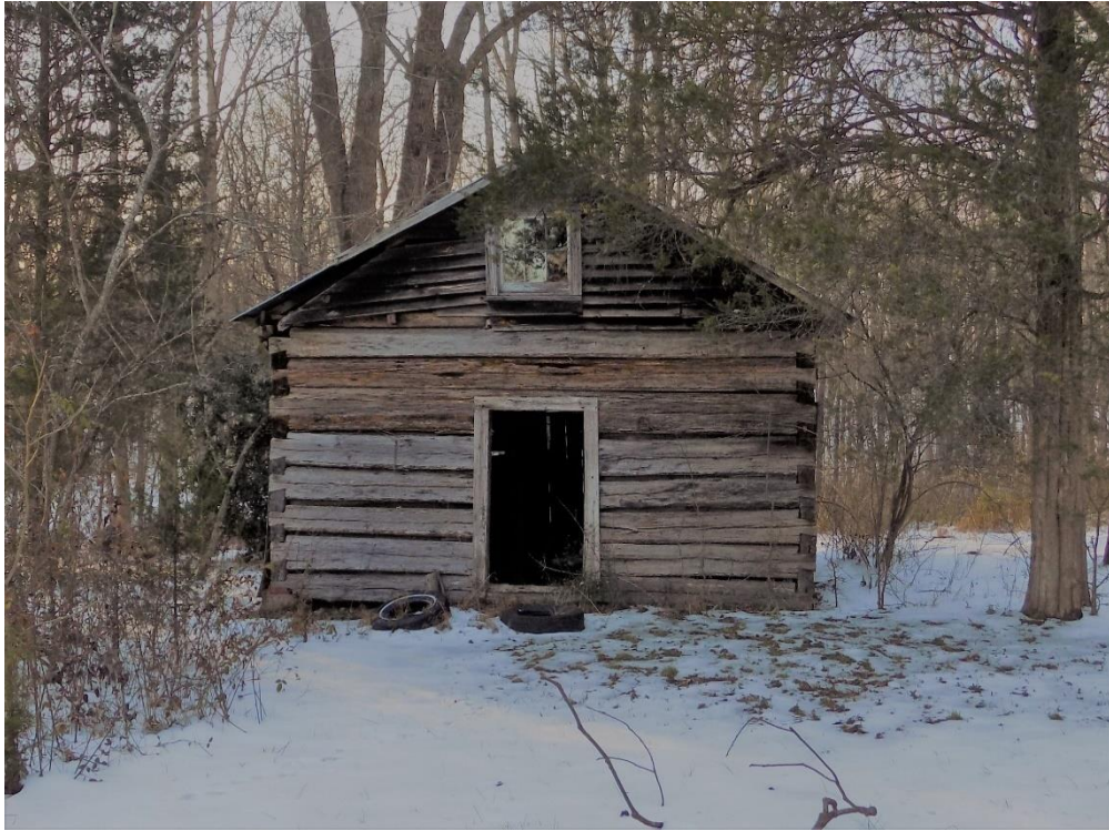
Façade of Sloop School, looking southwest
