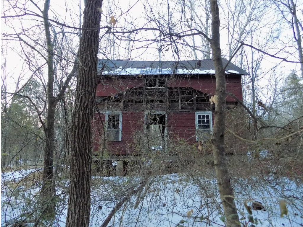
John Milton Faggert House (CA0388) façade, looking northwest
