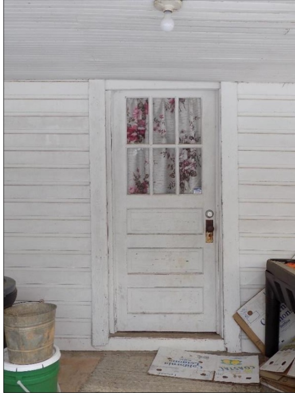
Single 3/panel, 6/light wood door main entry with drop siding and bead board ceiling
