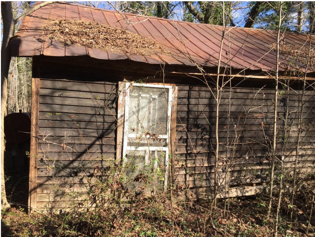
Weatherboard exterior and rear entrance to post office, looking north
