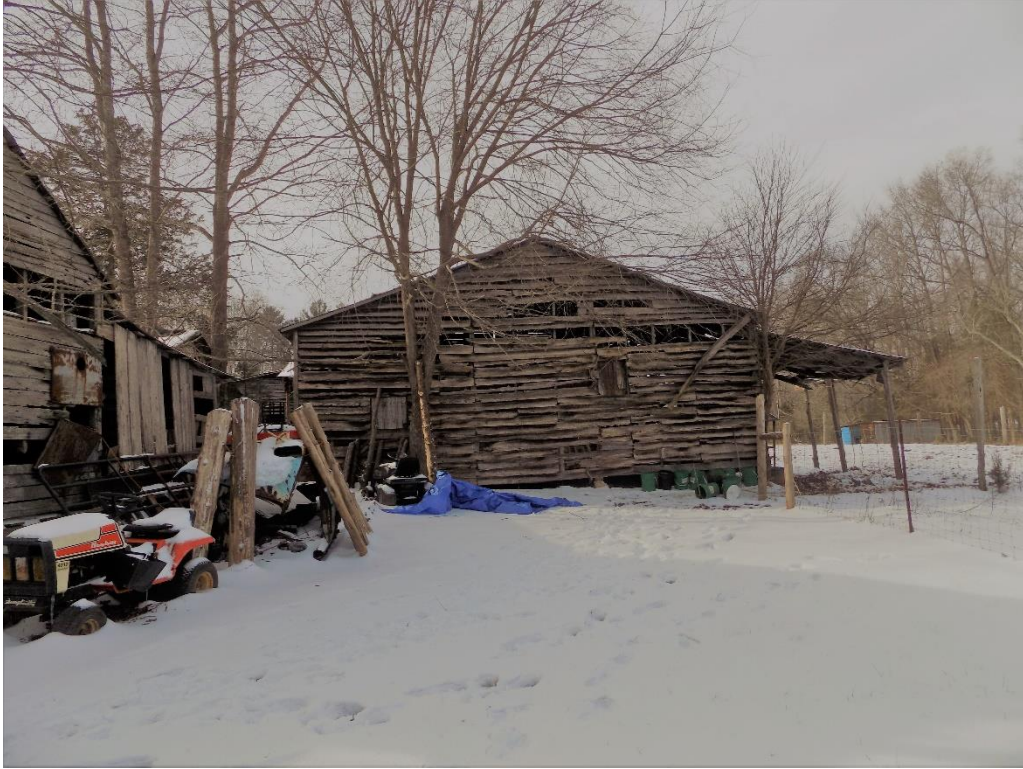
Rear elevation of the granary, looking west
