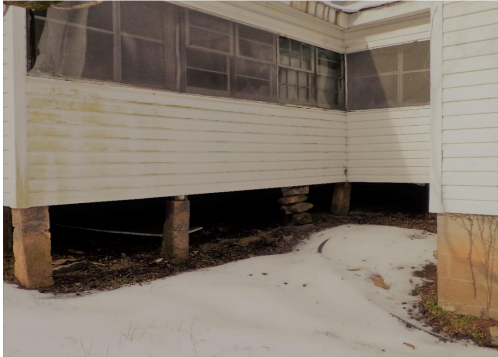
Granite pier foundation; rear shed porch
