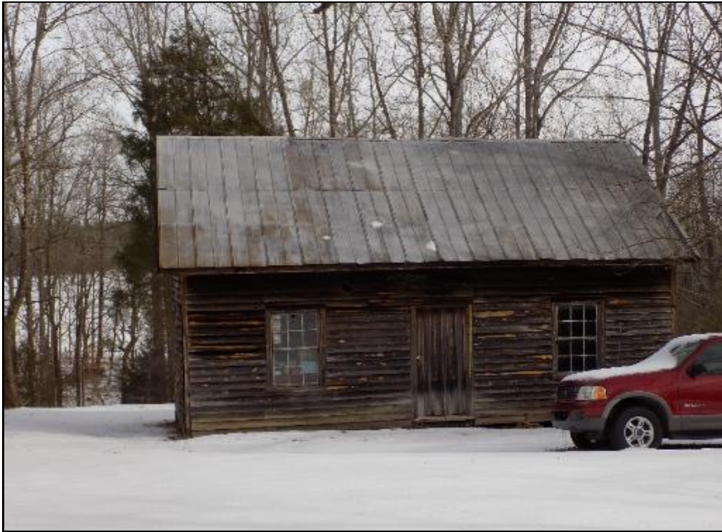
c.1850 frame smoke house, looking north
