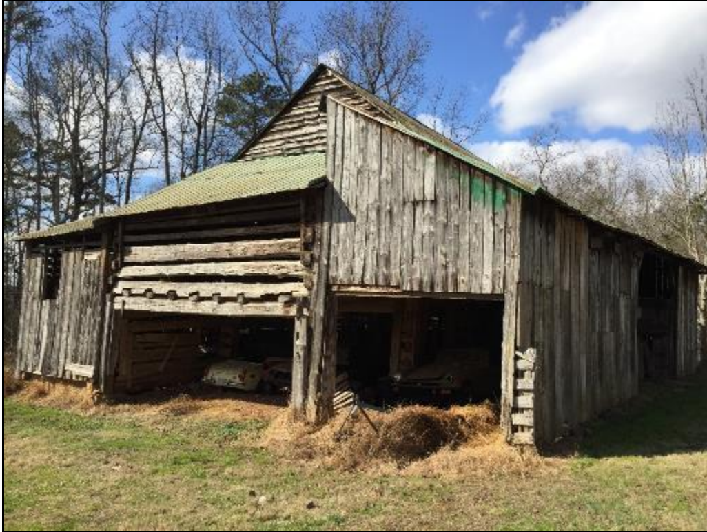
Log barn with frame additions; looking southwest
