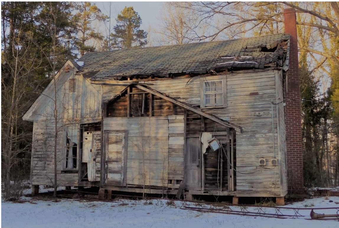
T. M. Yost house, rear elevation, looking north
