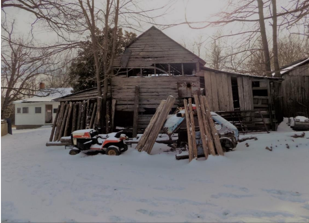
Rear elevation of tool shed, looking south
