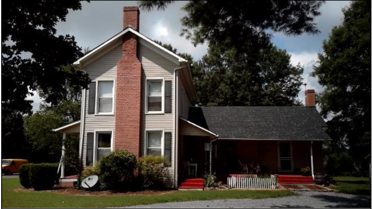
South elevation of Kever-Cansler House
