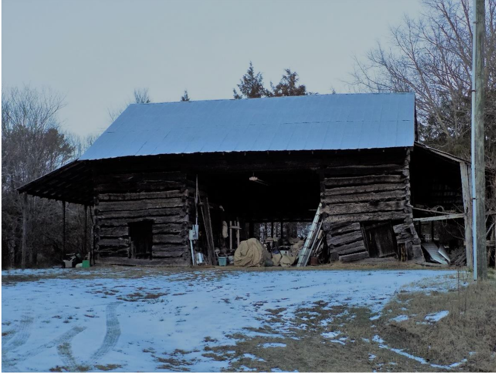
Double-crib log barn at John Milton Faggert property
