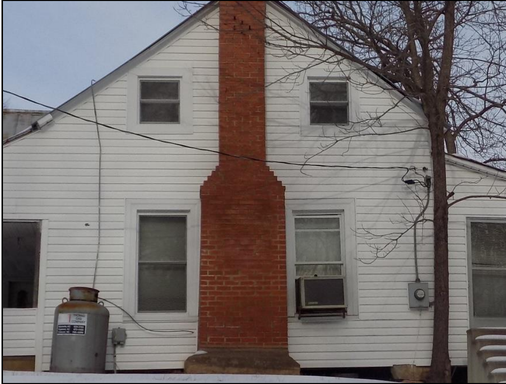
One-over-one replacement sash windows
