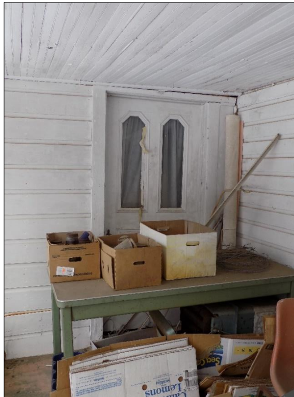
3/panel, 2/light wood door with molded trim; mix-matched drop siding
