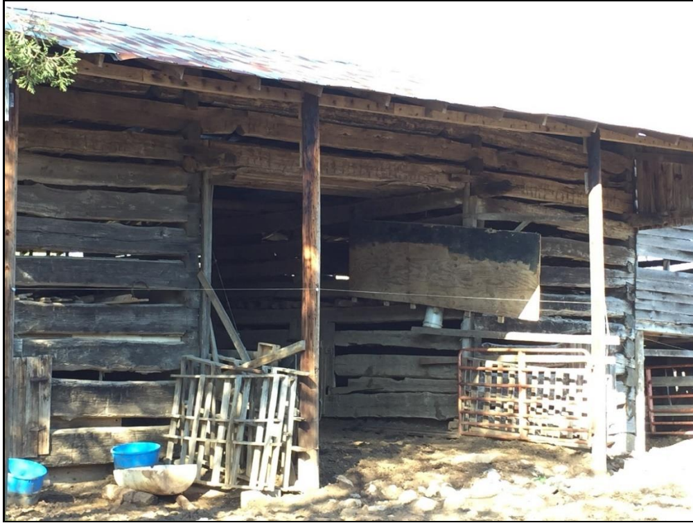
Central section of original portion of barn
