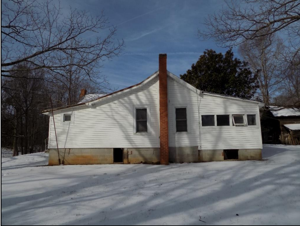
Rear (east) elevation of main house
