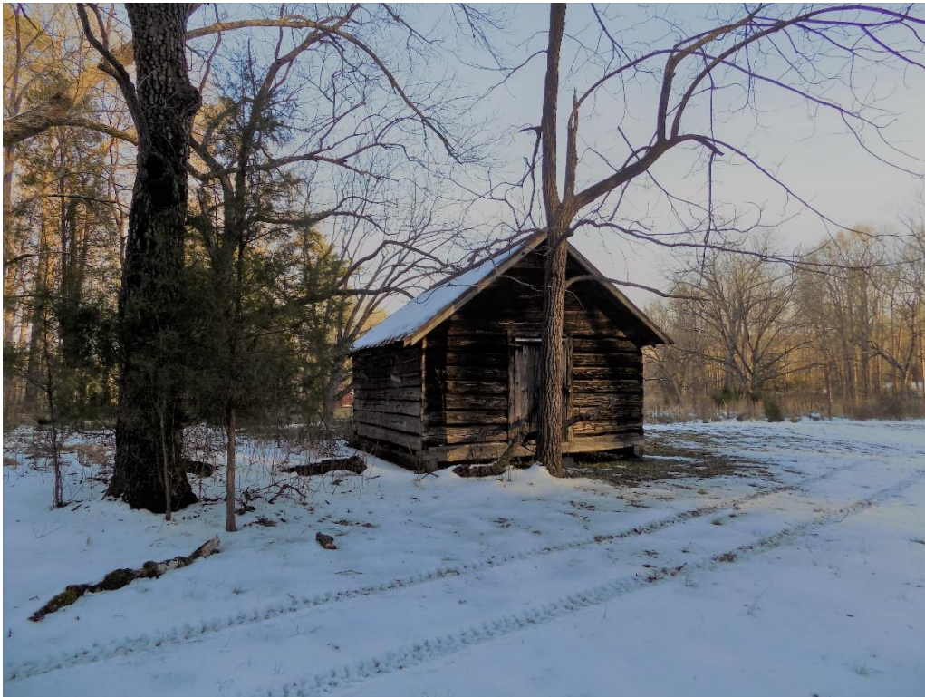
Log canning shed on southern parcel, looking east
