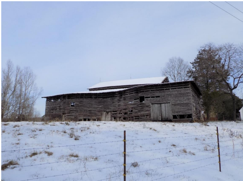
Rear (west) elevation of double-crib log barn
