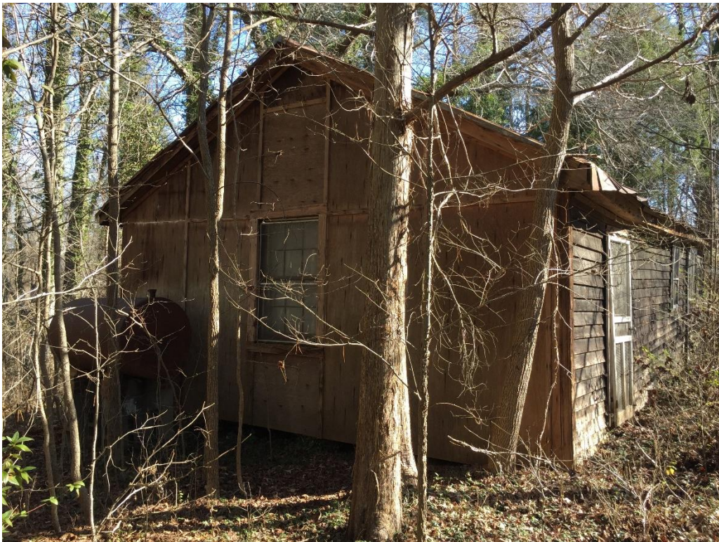
Rear elevation of post office with replacement siding, looking east
