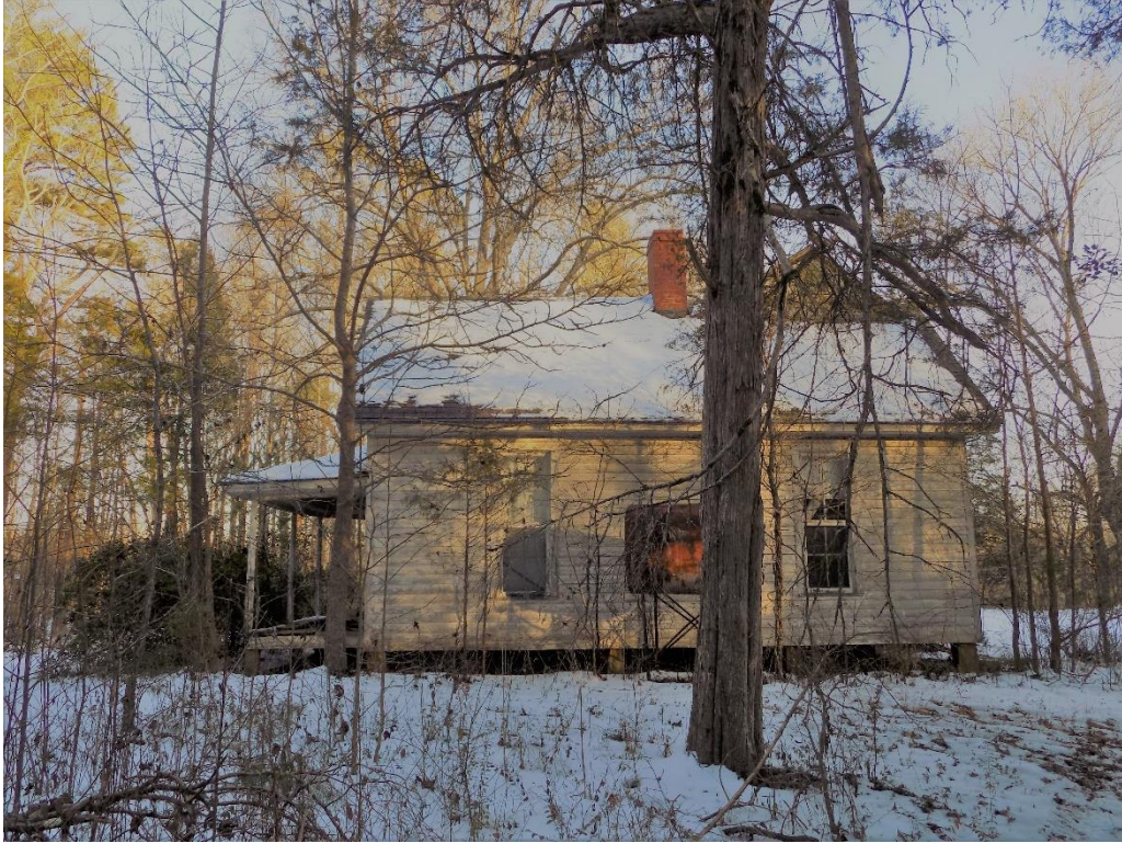
T. M. Yost home addition, looking east
